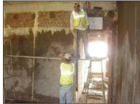
Adequate illumination levels in construction area
