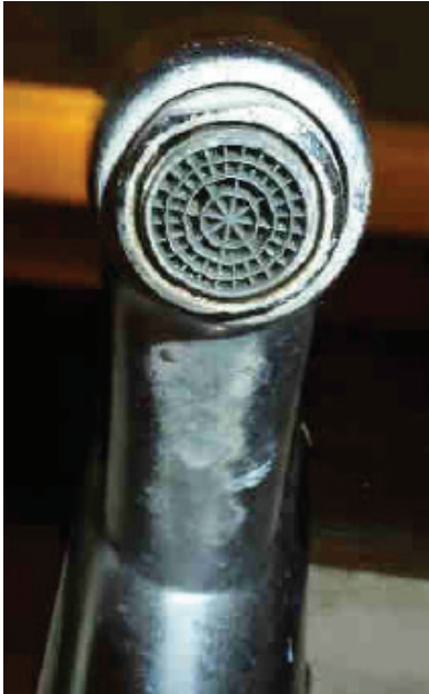
Aerators fitted to tap and dual Flush Cistern
