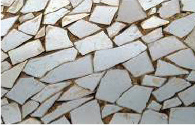
Roof covered with White paints
