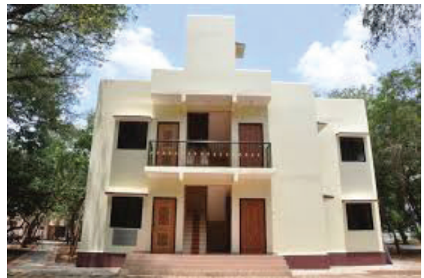
GFRG Demonstration Building – IIT Madras
