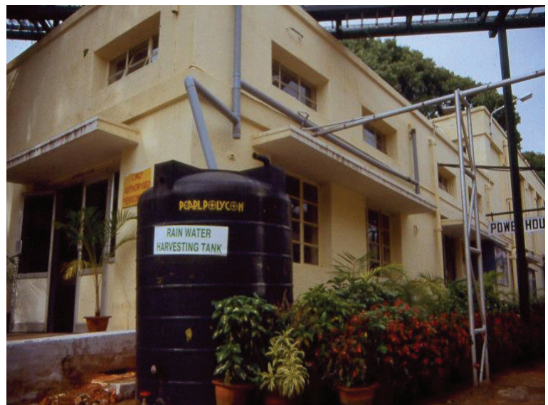
Roof top rain water harvesting tank
