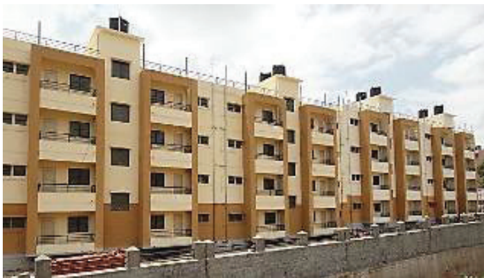
Monolithic Concrete Construction - BDA
