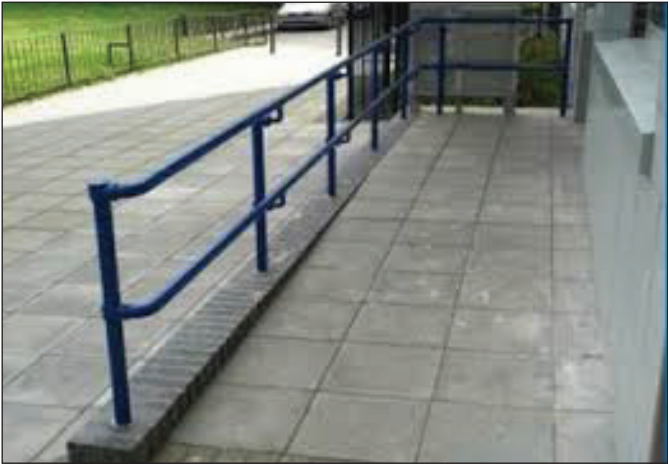
Non-slippery ramps with handrails
